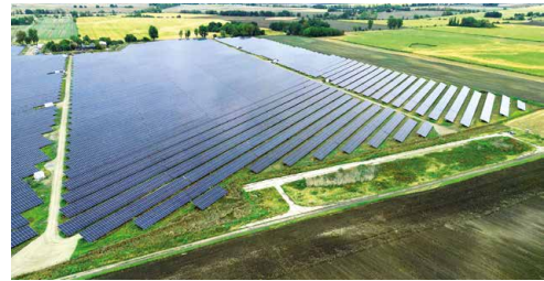
› Ground-mounted PV Letschin approx. 60 MW
